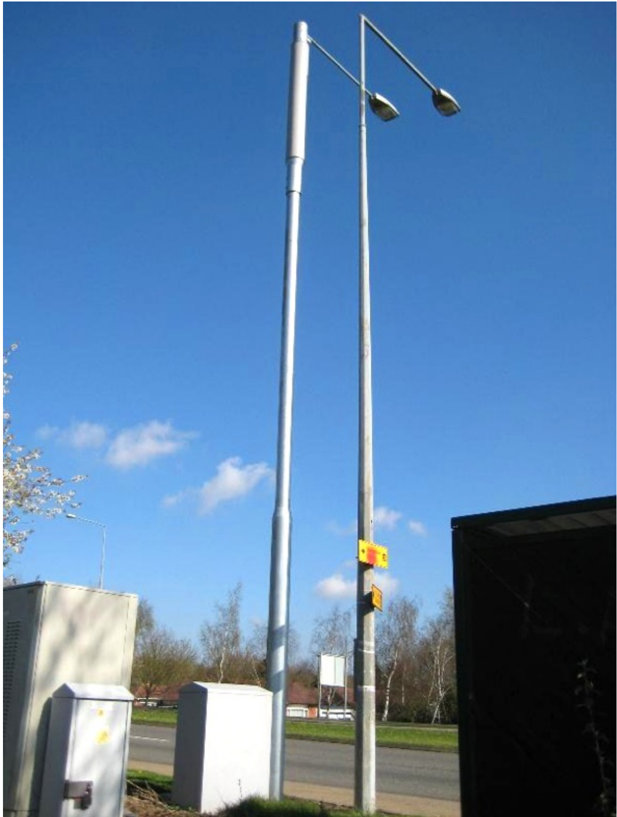
Cell tower disguised as lamppost, Milton Keynes, UK. Photo: Norfolk12.
