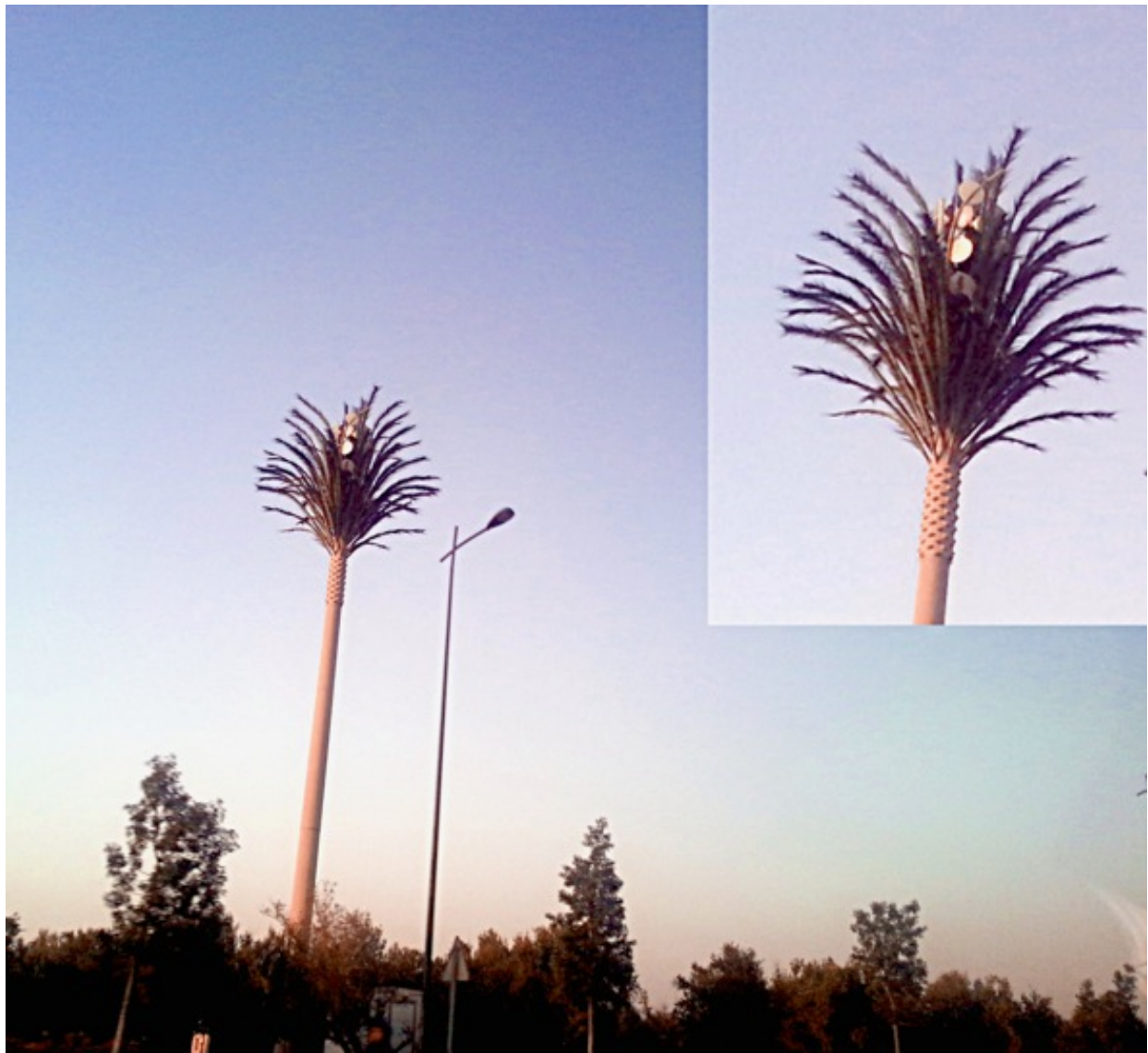
Cell tower disguised as palm tree, Marrakech, Morocco. Photo: Julian Oliver.
