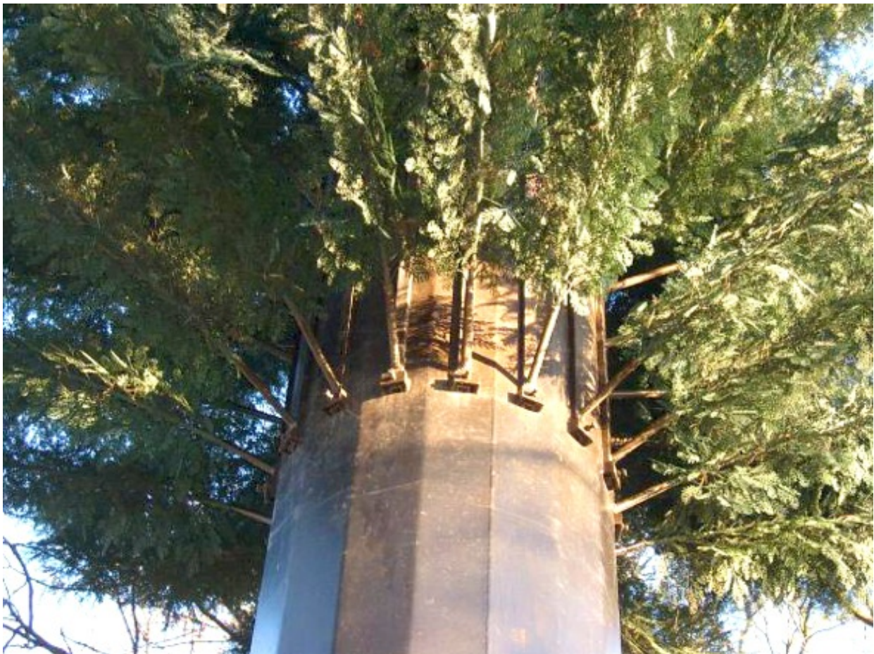
Cell tower disguised as fir tree, Bedfordshire, UK. Photo: Dragontree.
